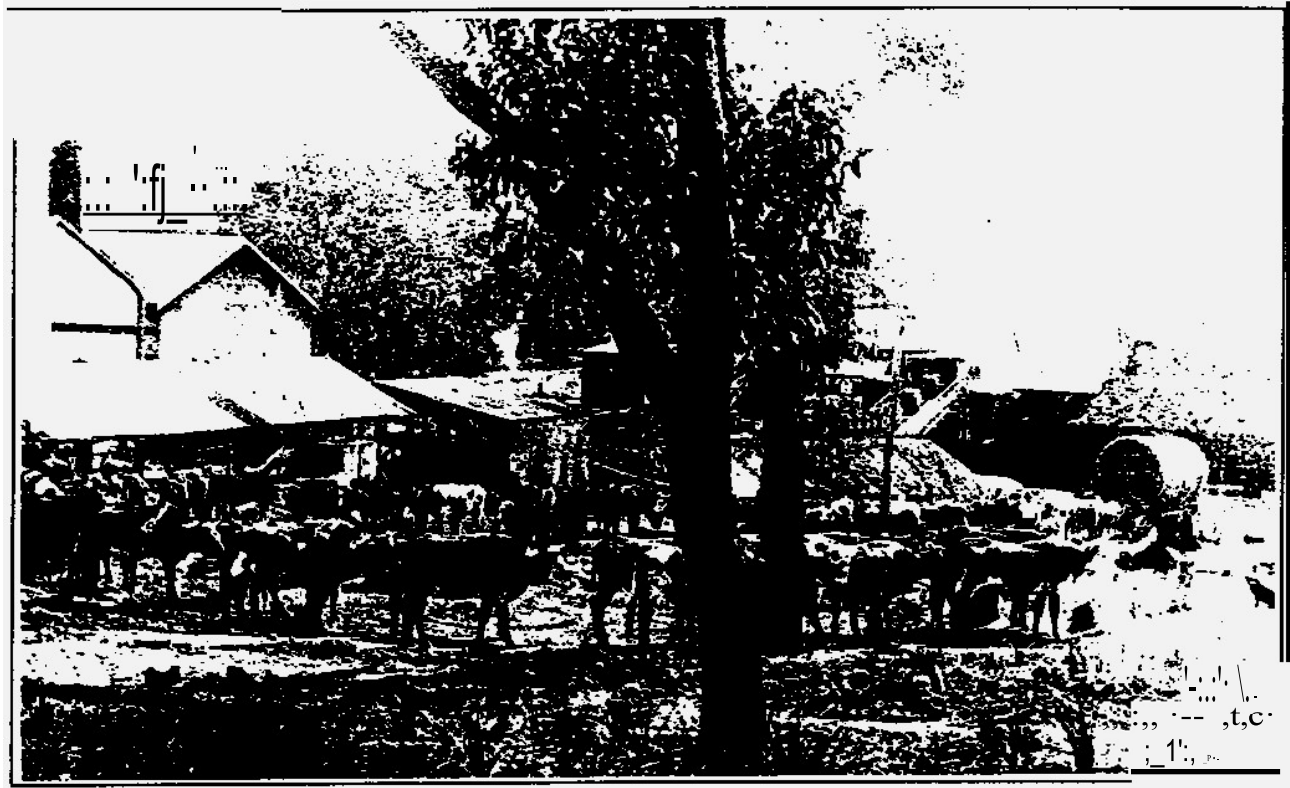
Bullock teams arriving at Wallarah Colliery's E pit around 1910 with a boiler hauled from Goninan's in Newcastle. By 1912 most of the company's plant was concentrated at E pit. Steam was generated by two Babcock & Wilcox boilers and two Cornish boilers. (source: A Beecham, Belmont, published in Newcastle Morning Herald 16 November 1983 p.20)
